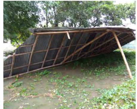
7. f) House construction material salvage
