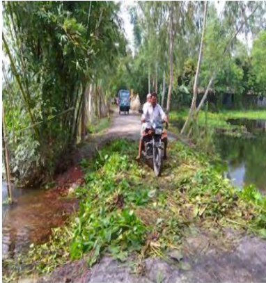
8. a) Road cutting for release of flood water and fill with hyacinth
