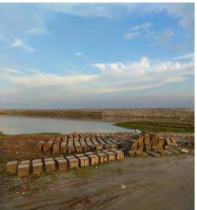
5. c) Teesta river revetment
