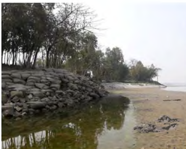
8. d) Erosion protection through sand bag
