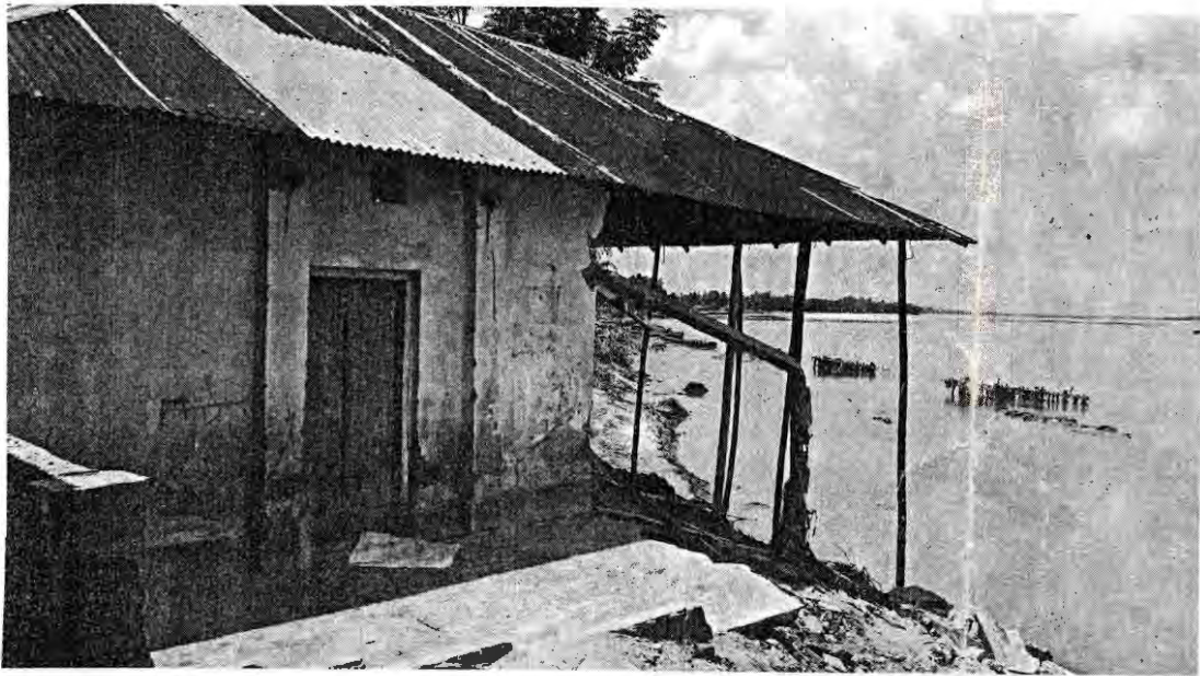
Like this mosque at Etapota village in Lalmonirhat Sadar upazila, many set-ups including dwellings are under the threat of erosion by the Dharla river during the ongoing recession of floodwater.
