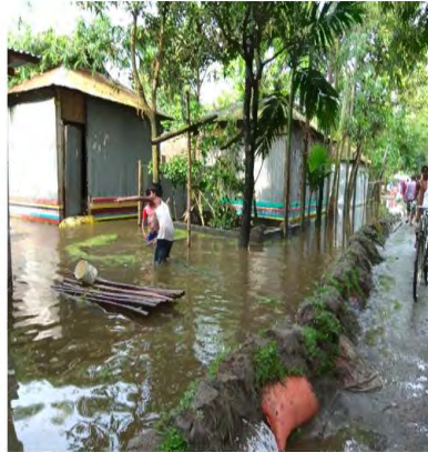
8. b) Artificial levee construction to prevent flood water
