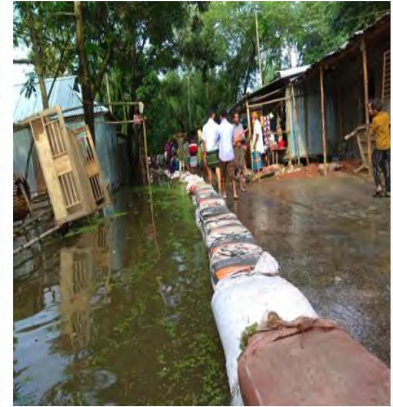
8. c) Sand bag piling for flood protection
