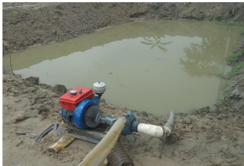
Plate 3.5: Pond excavation in the study area
