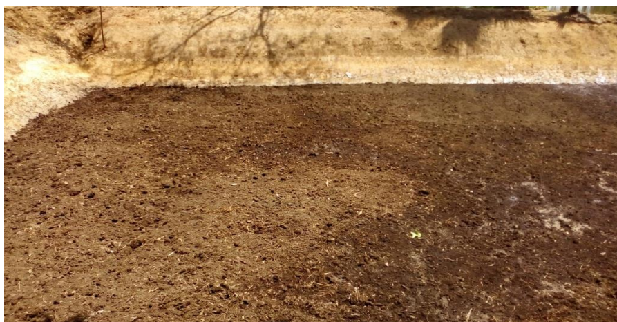
Plate 3.8: Pond excavation in the study area
