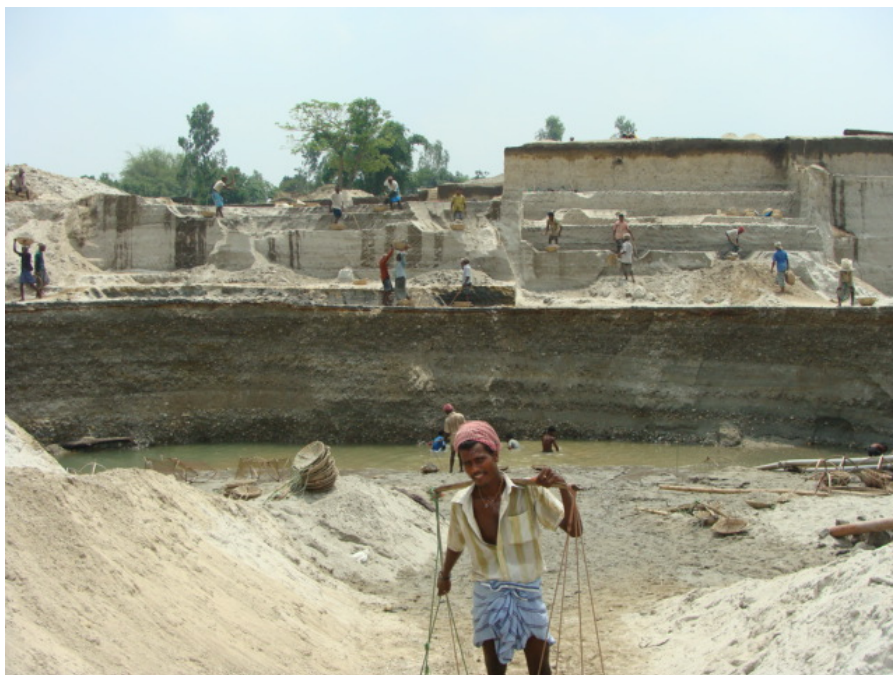
Picture 4: Elimination of Top Soil from the Land
