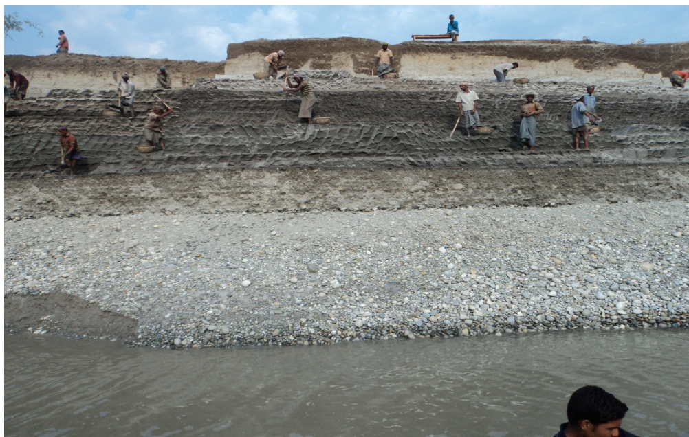
Picture 1: Process of Underground Stone Collection in Panchagarh District
