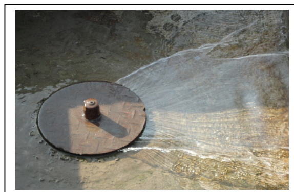
Photo-10: Water uplifting from DTWs
