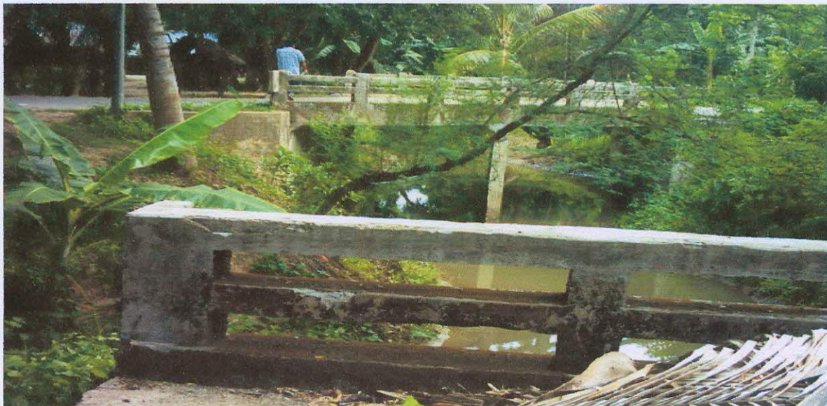
Plate 15: Two culverts were constructed within two years and located at the same point; the photograph was taken from old one
