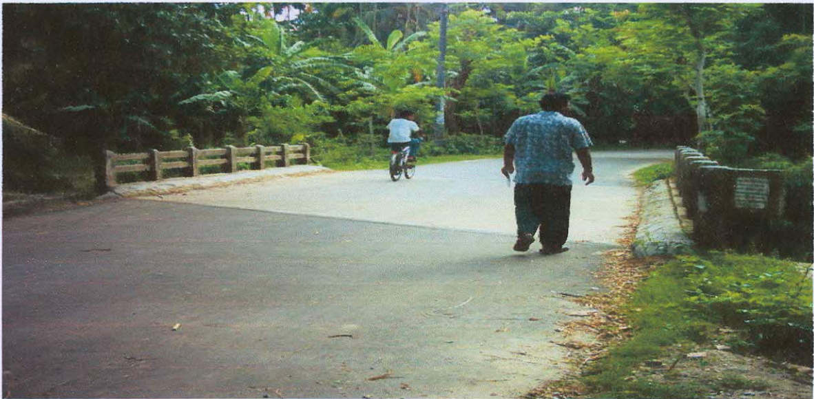
Plate 14: Culvert constructed by LGED and CARE in 1995
