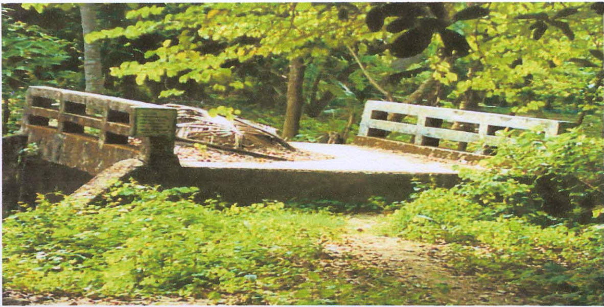
Plate 13: Culvert constructed by the fund of Relief and rehabilitation ministry in 1993
